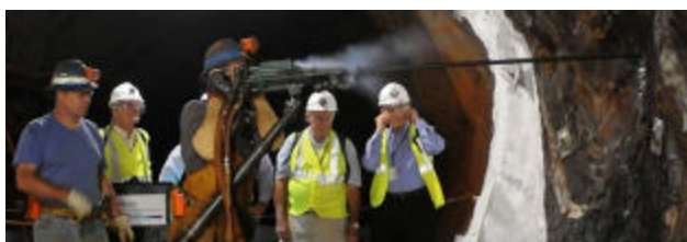
Technician Bill Heisinger drills holes in the shaft wall for a plaque June 22 in a dedication ceremony the Sanford Underground Science and Engineering Laboratory at the former Homestake Gold Mine in Lead, S. D. Before the labs are built, crews must also stabilize the tunnels and install new infrastructure.
